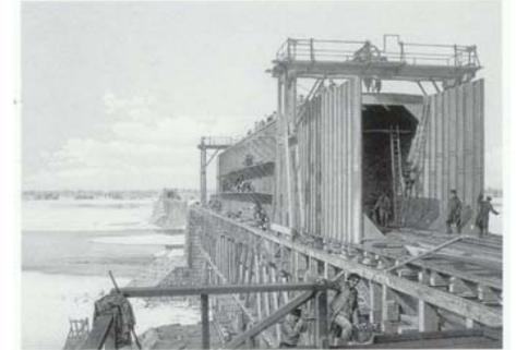
Victoria Bridger tubes under construction on travelling gantry
